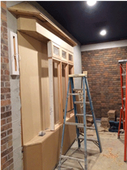
Old Lunden theme home theater lobby, construction.
